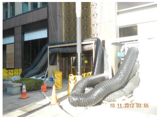
写真-2 Wall St
